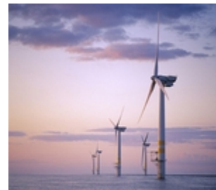
The 3.6-megawatt wind turbines of the Arklow Offshore Wind Farm in the Irish Sea near Arklow, Ireland. Bloomberg News
